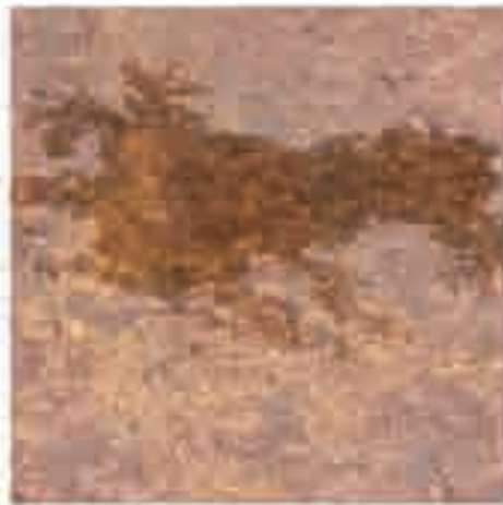
Unprotected pavers will allow UV, dirt and chemicals to penetrate the surface, causing color to fade and the surface to breakdown.
