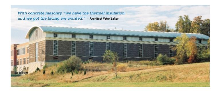
building's wall would show an exterior face shell 1.5 inches (38 mm) thick, a one-inch (25.4 mm) cavity for water drainage, two inches (50.8 mm) of rigid insulation for thermal performance and three inches of grout. Builders installed cabling and conduits in the cavity between the insulation panel and the 1.5-inch-thick interior face shell, then filled the remaining space with 3,000 psi concrete grout.
