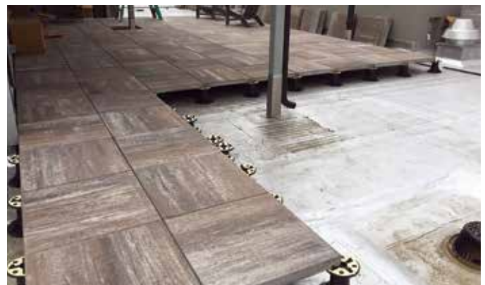
Example of roof deck under construction.
