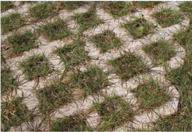
Grass Pavers Installation Pattern
