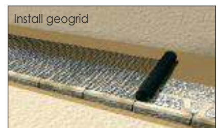
Install first course of pattern on top of geogrid
