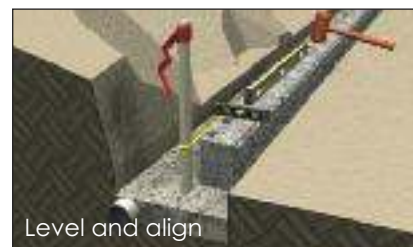
Install facing unit
